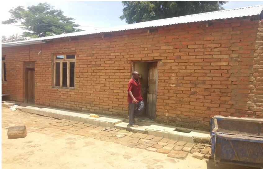
Figure 2: Mr Mlowe poses in a photo at his house after renovating. Photo Credit: Dr Didas Kimaro
